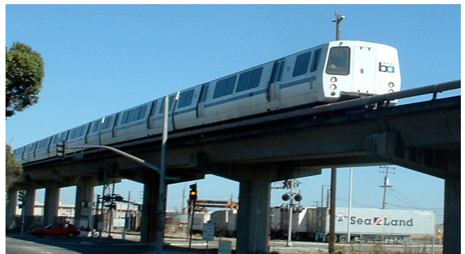
Figure 4 BART Train on Elevated Track
